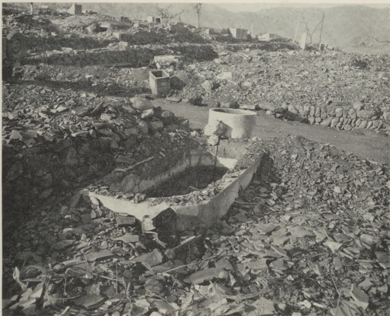
Photo 16. Small water tanks for fire fighting, made of dirt and plaster, built by some families. Concrete water receptacles, 40 to 70-gallon size, may be seen in background.
